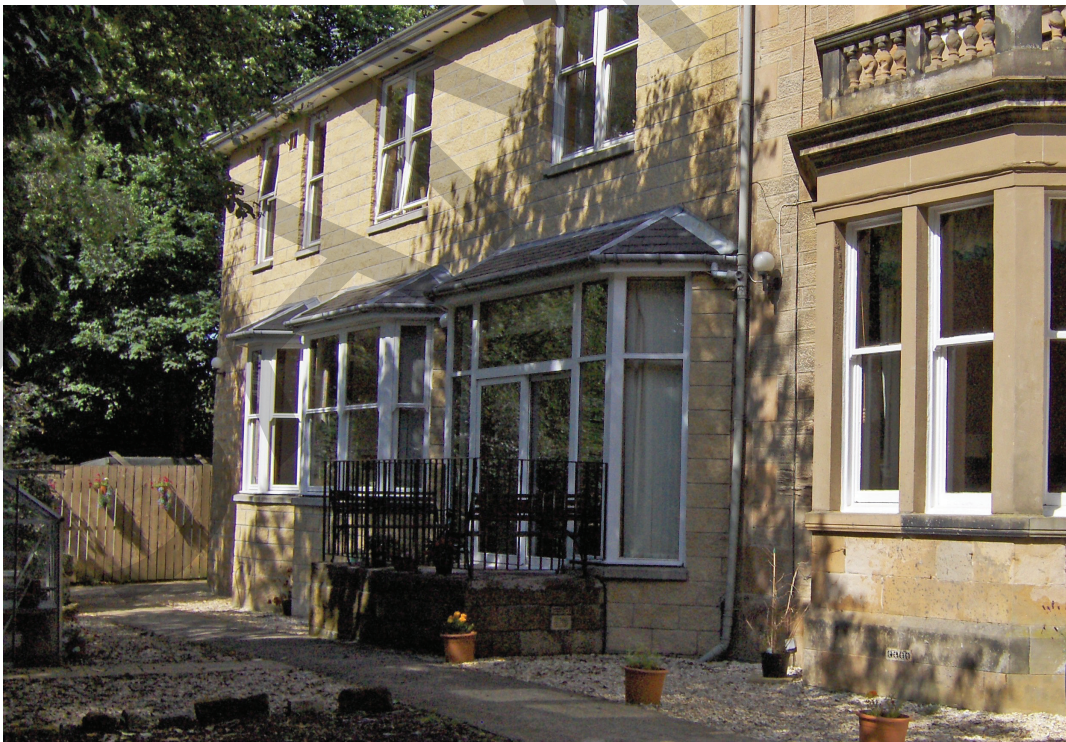
Trees can block direct sunlight: a care home in Scotland. Photo: Annie Pollock
