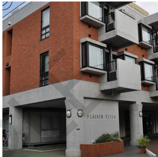
Fig. 17 The home is a three-storey reinforced concrete structure, which houses 60 residents of which around 20 residents currently require care for dementia
