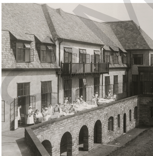
Fig. 2 Balcony at the Elsie Inglis Memorial Pavilion, Edinburgh, c. 1935
