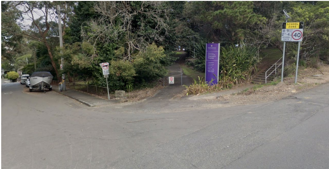
Photo 4 – Poor Condition Footpath – South / Western Corner of St Vincents Road Intersection with River Road
