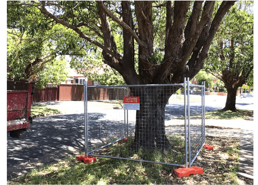
Figure 3 – Example of temporary tree protection fencing
