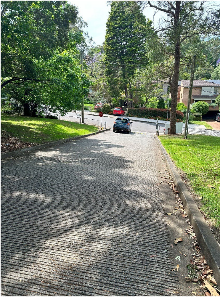
Photo 5 – Steep Driveway Access
