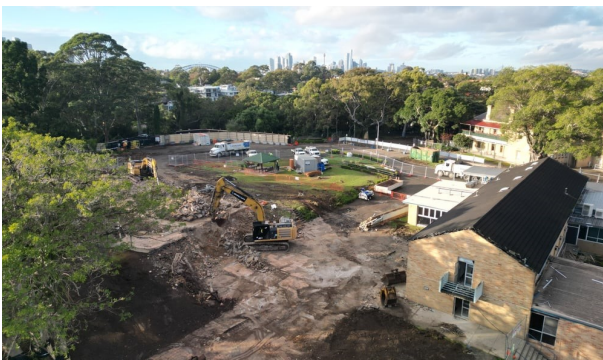
Early demolition works begin
