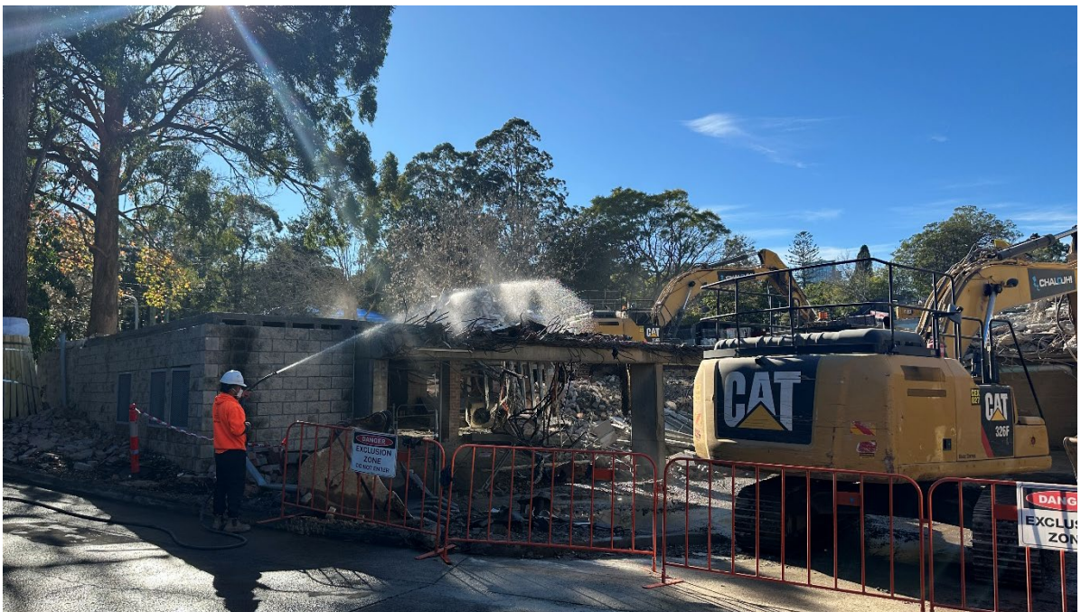
18. Implemented dust control measure near the active demolition work zone. 23/06/2026
