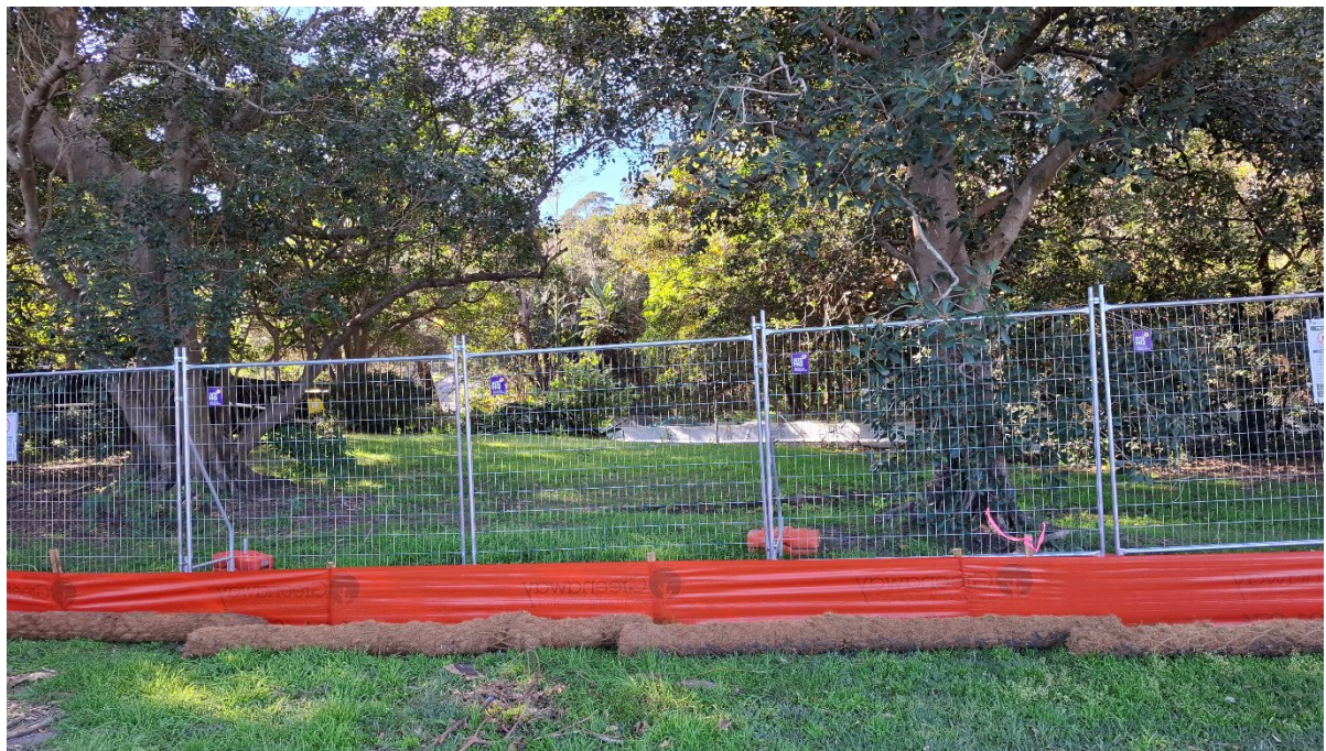
10. Implemented tree protection and erosion and sediment control measures. 23/06/2026
