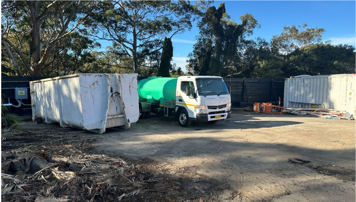
23. Large waste skip bin and water truck in the eastern part of the construction zone. 23/06/2026
