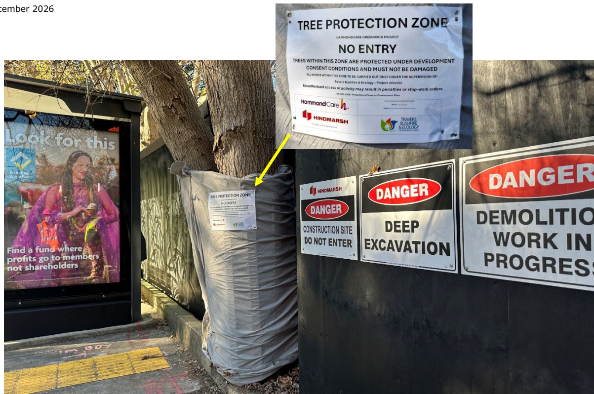
9. Construction site signage on the hoarding near the River Road bus stop. Implemented tree protection measures and Tree Protection Zone signage. 23/06/2026
