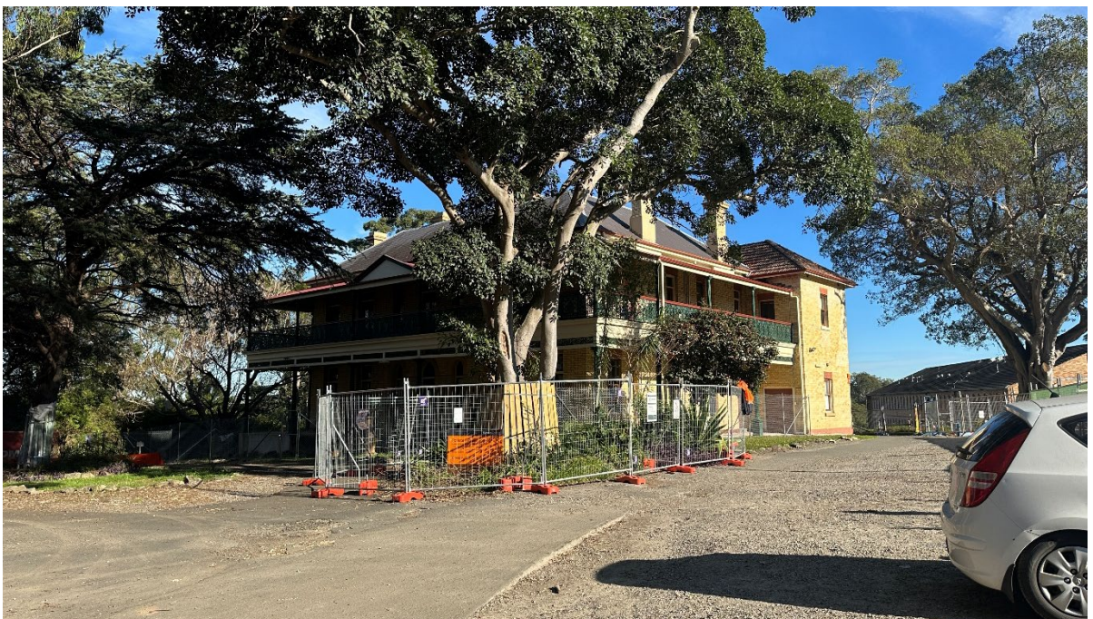
12. Implemented tree protection measures around a tree located near Pallister House. 23/06/2026
