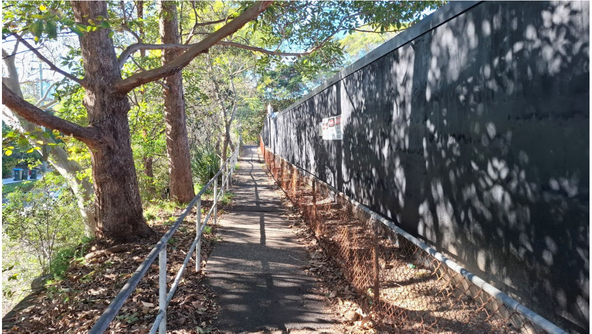
7. Looking east along the River Road footpath from near the Gate 2 (or H2) entrance. No obstructions on the public way. 23/06/2026
