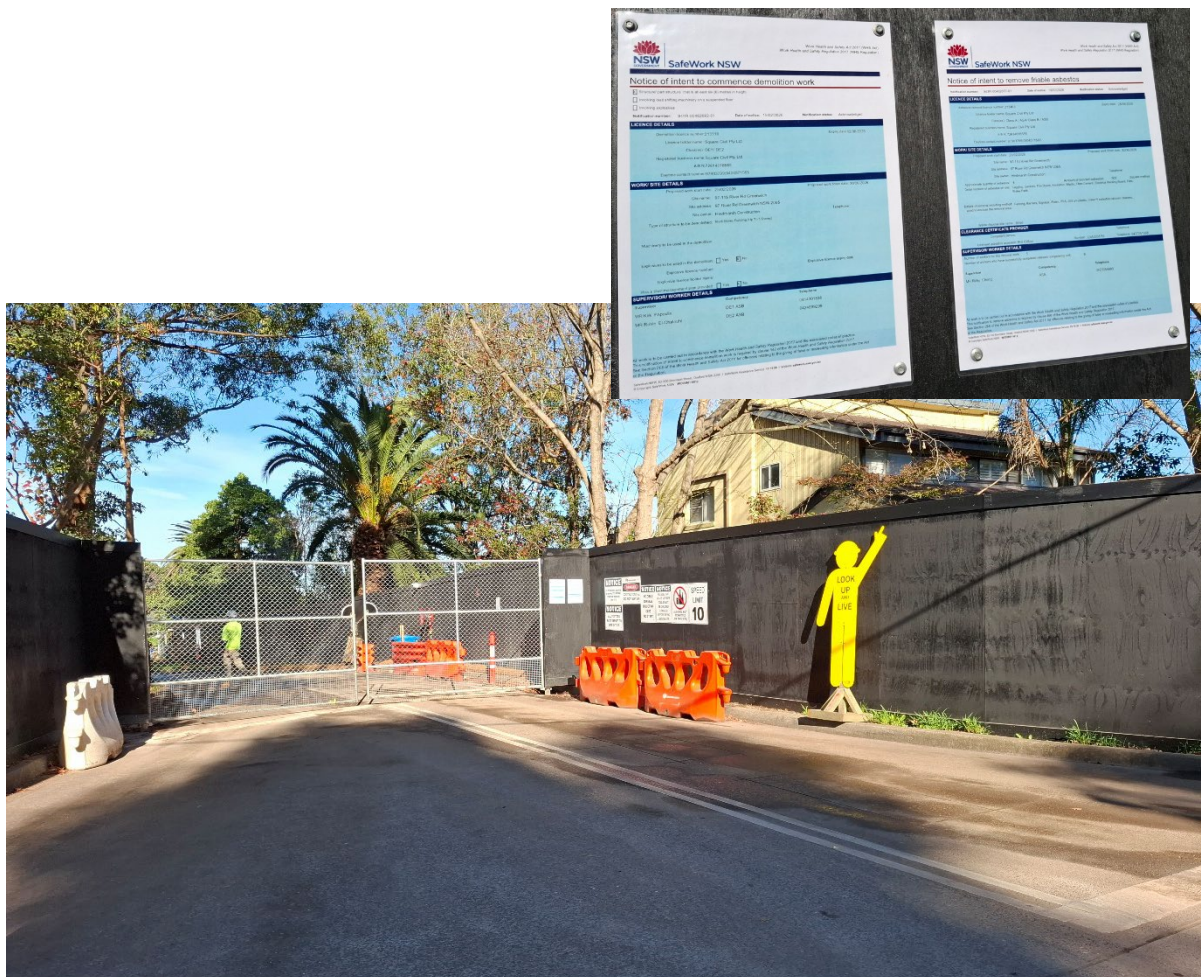
2. Gate 1 (or H1) entrance from River Road. SafeWork NSW Notices posted to the right of the gate. 23/06/2026
