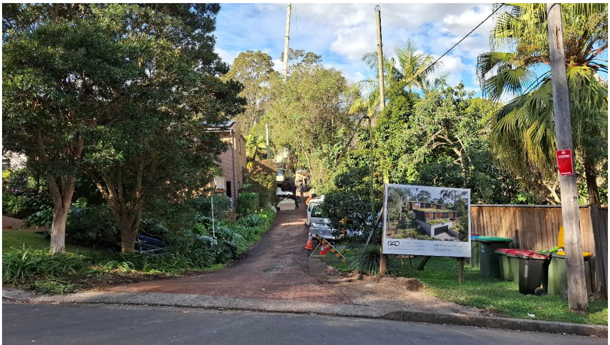
20. Construction work being carried out at 22 or 24 St Vincents Road. 23/06/2026
