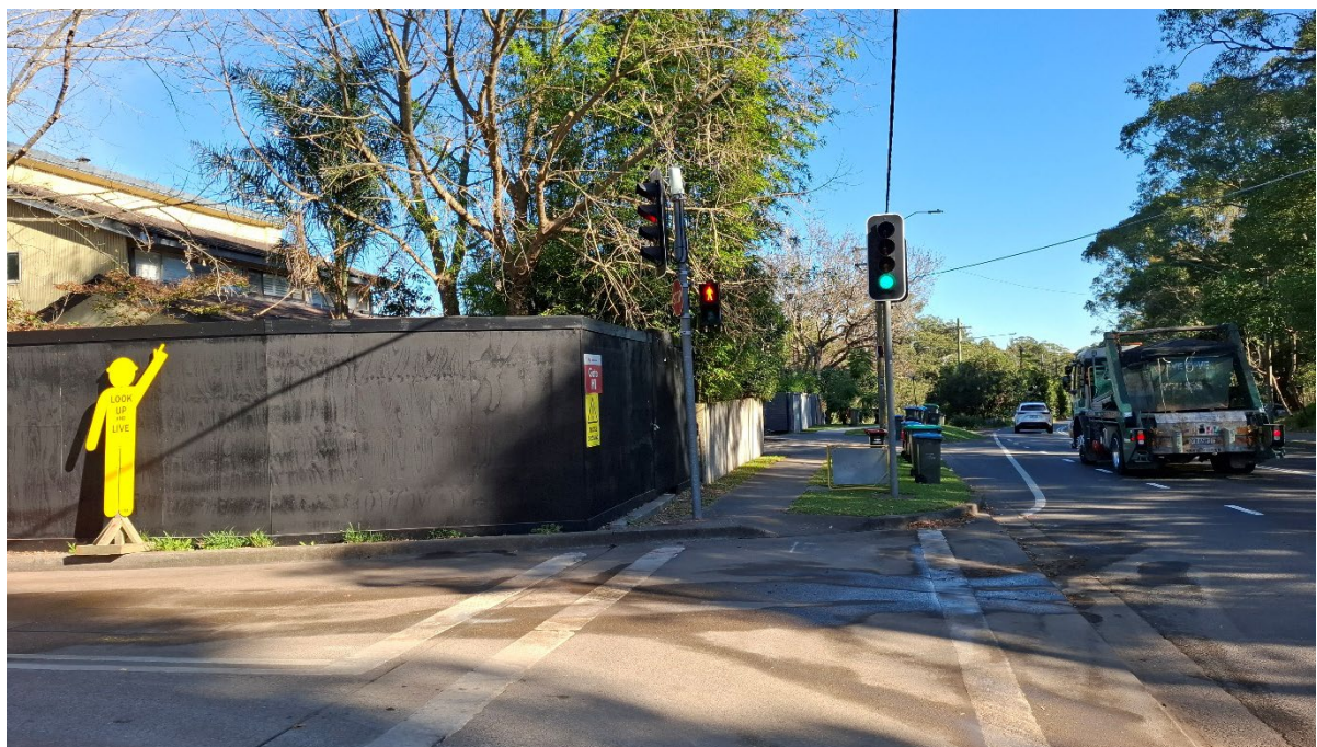
4. Looking west along River Road from the Gate 1 (or H1) entrance. No trucks queuing or obstructions or evidence of tracking of dirt onto the public way. 23/06/2026
