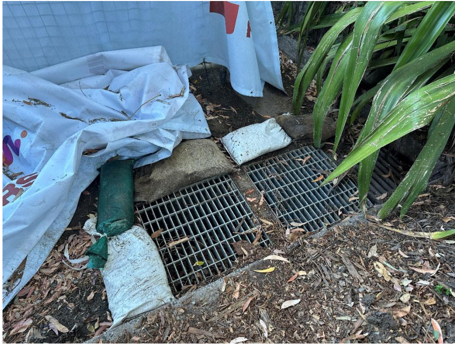
Photo 3: Sediment controls used around a stormwater drain located within the south eastern portion of the site.
