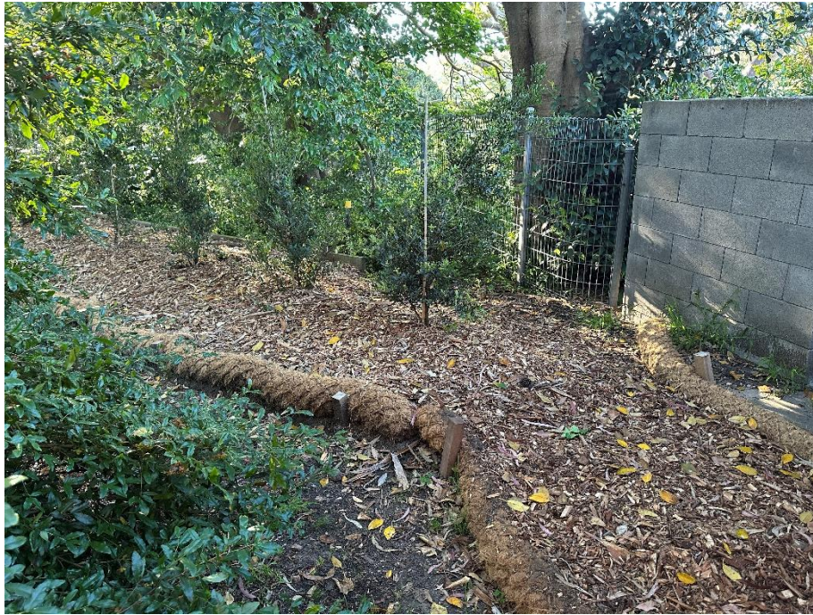
Photo 5: Sediment controls along the southern boundary of the site, looking to the south.
