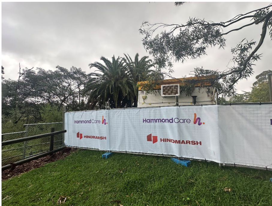
Photo 2: Fencing installed around the site offices within the south western portion of the site, looking to the west.
