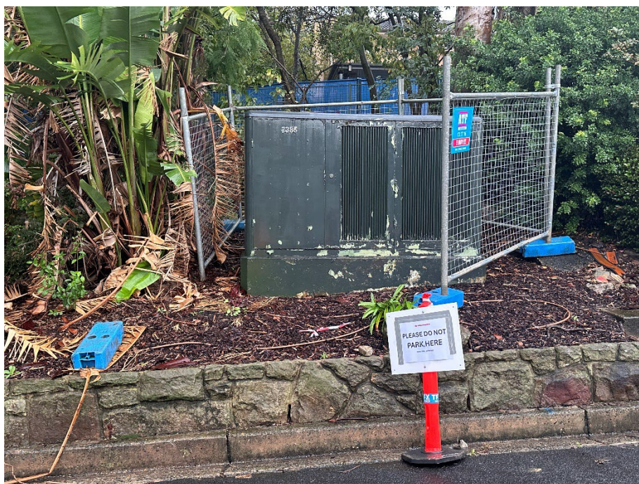
Photo 7: Fencing installed around the substation as part of Stage 1 construction works.
