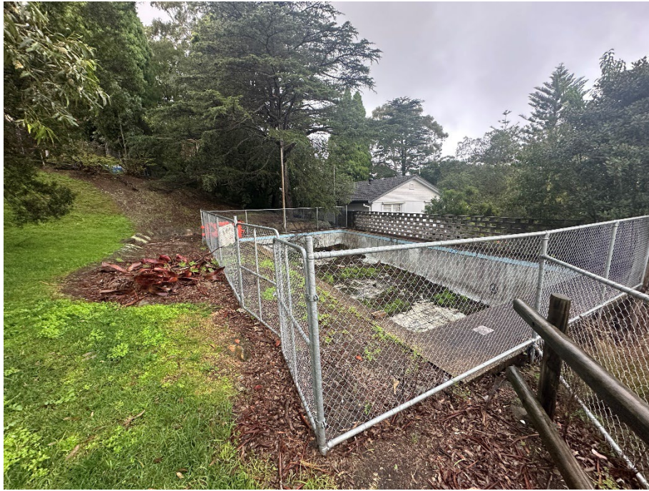
Photo 3: Fencing installed around the former pool to be filled in as part of construction works, looking to the south east.
