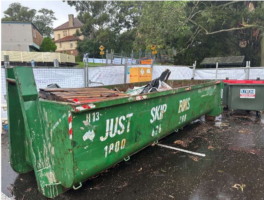
Photo 1: Waste collection area located adjacent to the site offices within the southwestern portion of the site, looking to the north east.
