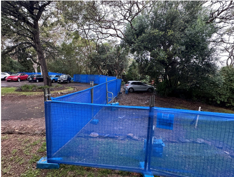
Photo 9: Fencing installed along the southern boundary, looking to the east.
