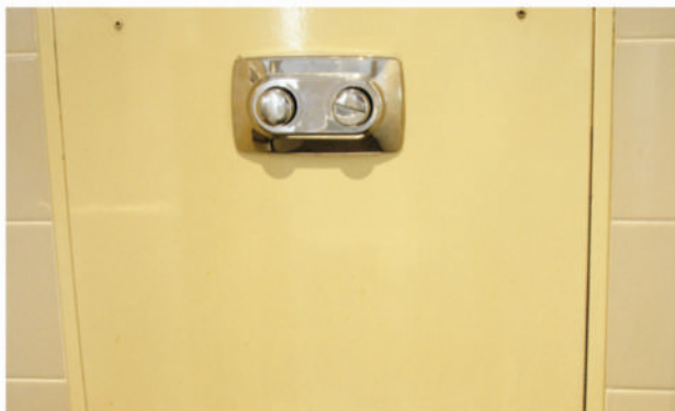
Cistern behind a fascia, with low contrast, buttons set high and ones that are hard to push—a range of design issues to avoid.
