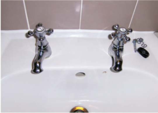
These familiar cross head taps are in a care home for people with dementia.
