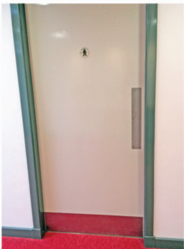
This sign is too high for most people let alone older people.
