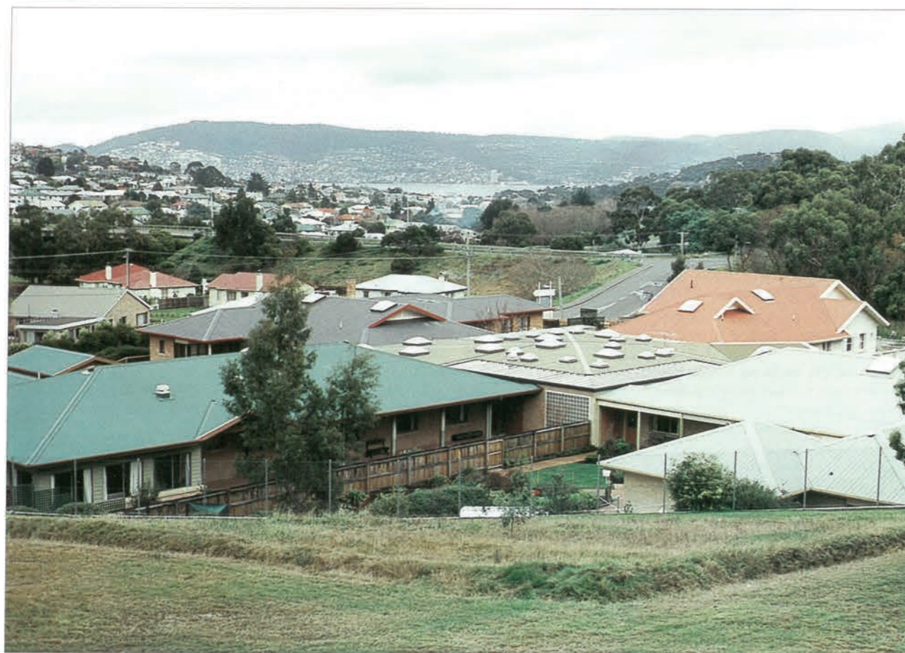
The ADARDS nursing home: A view of the buildings showing the steep site. Note the skylights which allow extensive use of natural light.
