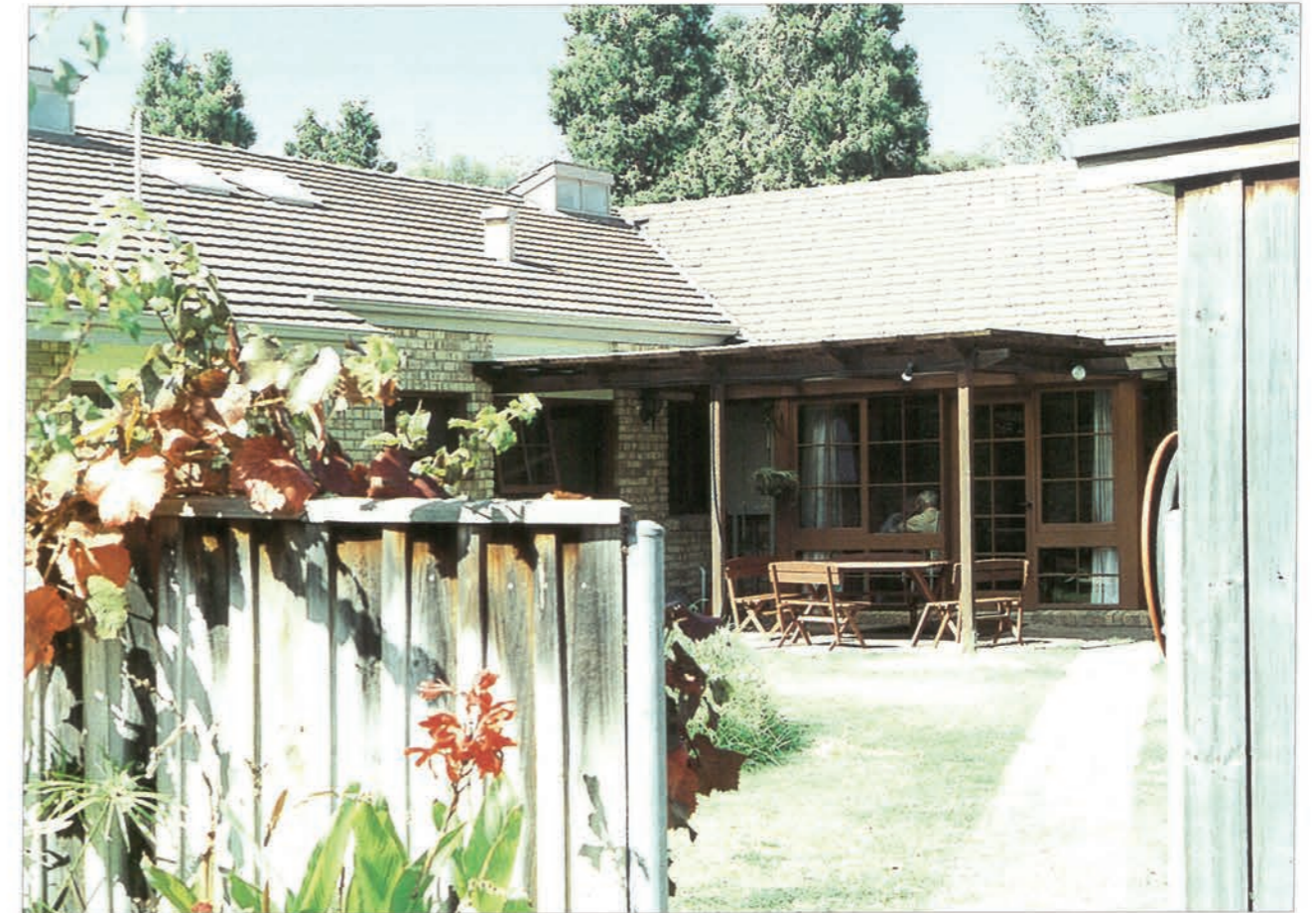
The secure rear garden with terrace and enclosing fence is an essential element of the design.
