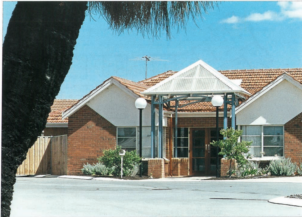
The main entrance. Kinross Hostel is part of a complex of dementia-specific facilities.
